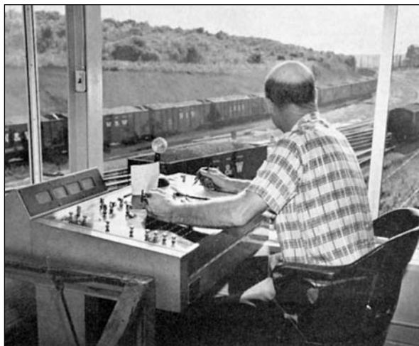
Car retarder Operator W. L. Bentley operates the remote controls governing the movement of loaded coal cars into the new classification yard.
